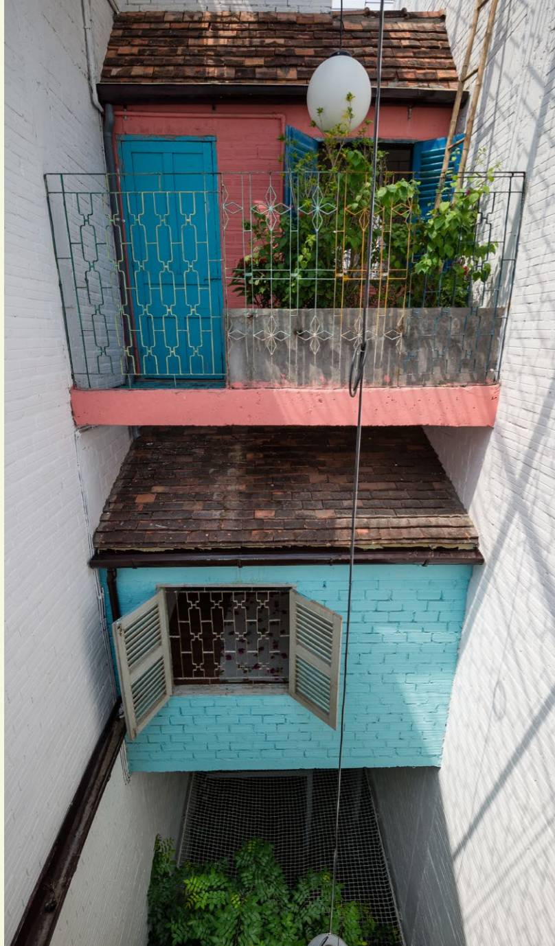
Above Finishing materials like indoor roofing, windows, and doors were salvaged from demolished homes.
