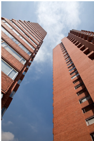
01 View of the towers from below 02 Tower C of Bogotá's iconic Park Towers
