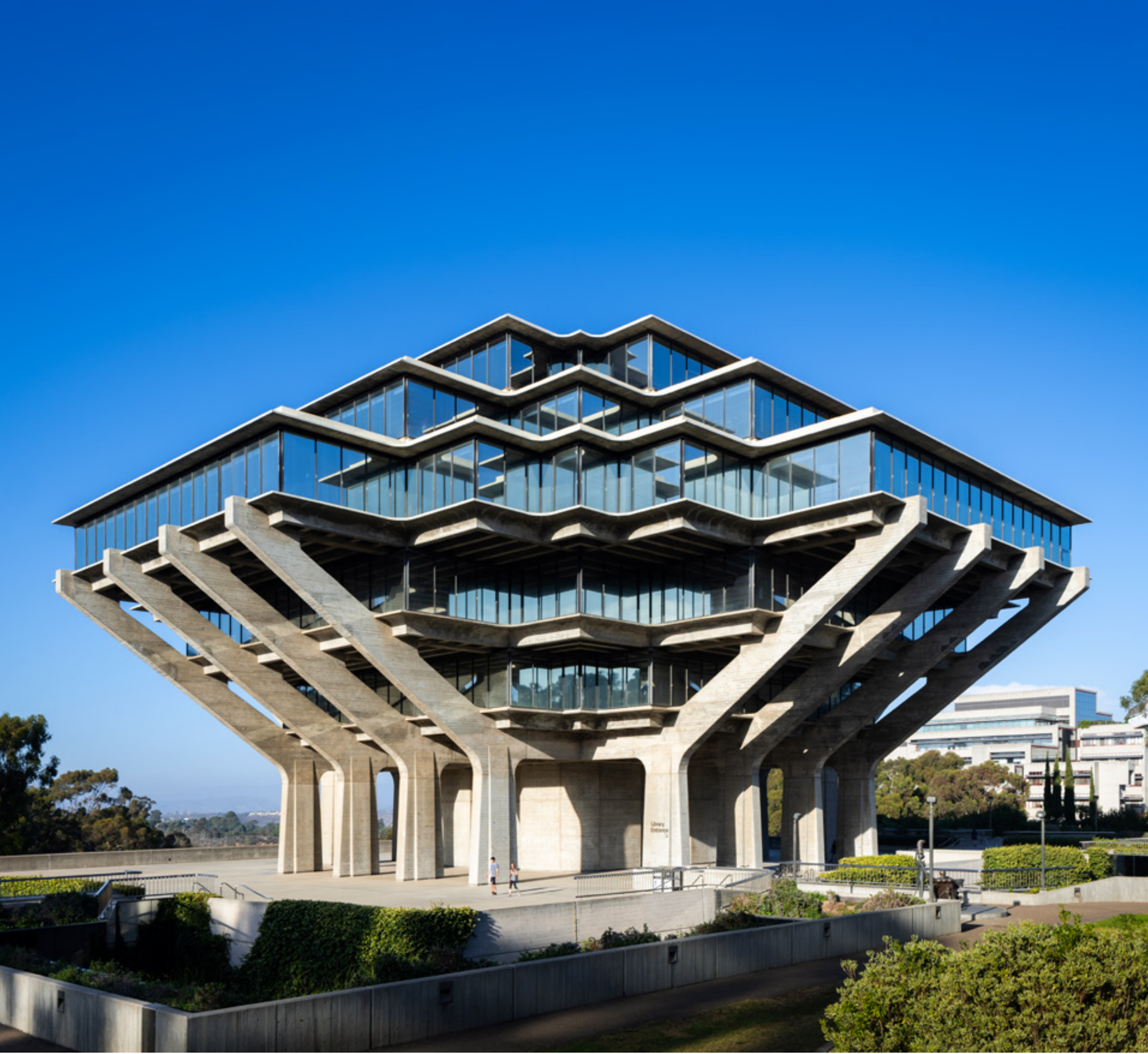
Curved concrete columns support the stepped, glass-clad structure—which rises above a plaza and sunken courtyard—like outstretched hands.
