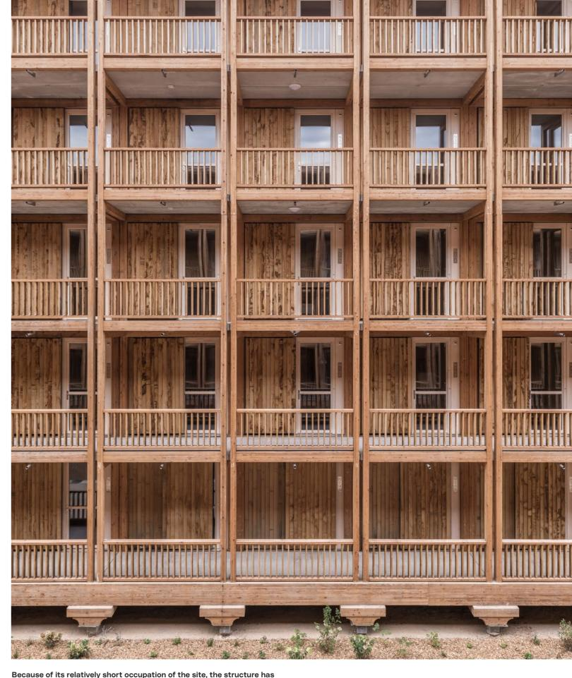
Because of its relatively short occupation of the site, the structure has been designed to touch the ground lightly, ensuring that after the building has been removed the site can regenerate. Using a "dry" construction on timber piles reduces the impact on the surroundings both during and after construction, safeguarding the ecology of Rigot Park.
