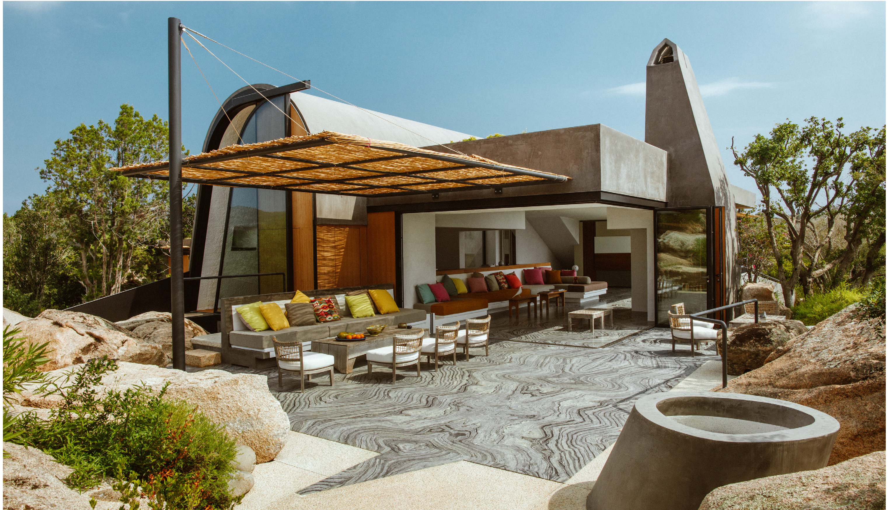
Sliding windows open up the living space to the terrace with marble floors flowing between the two.
