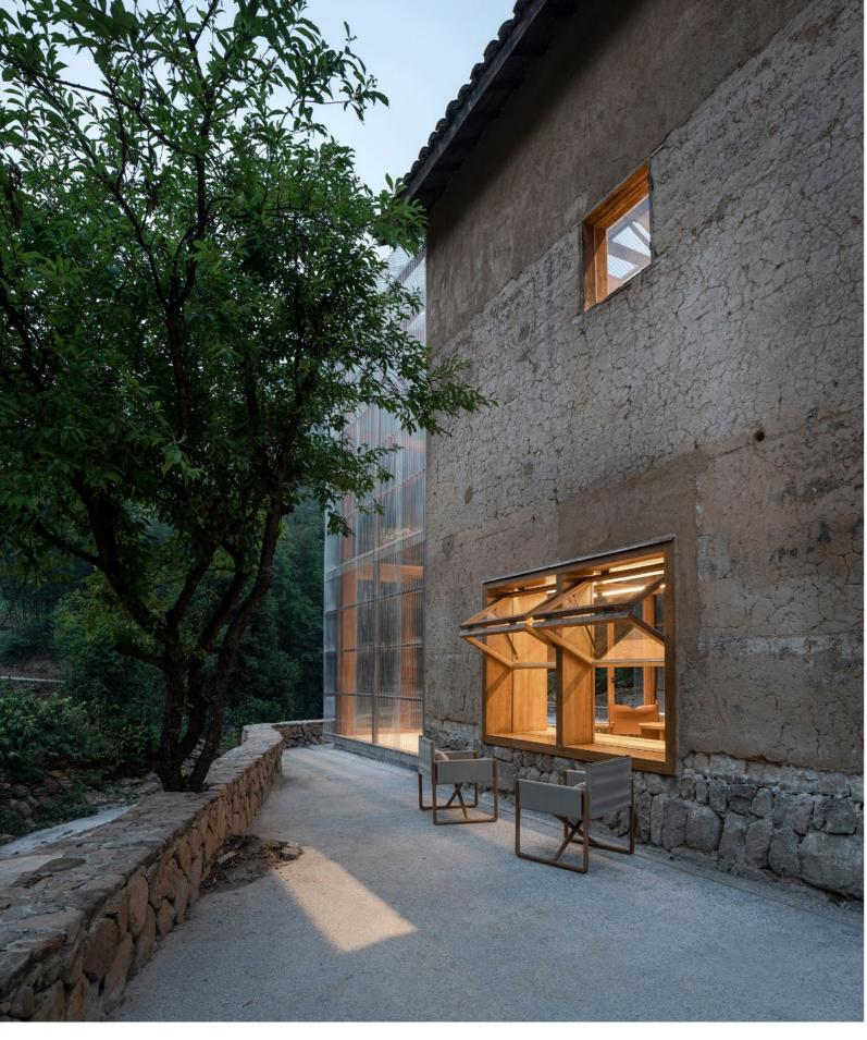
Removing the internal partitions of the existing 7 m-tall (23 ft) barn reduced the existing structure to a skin, into which new openings have been made to better serve the activities taking place inside. These glazed insertions give a sense of lightness to the old building, which appears to glow from within at night.
