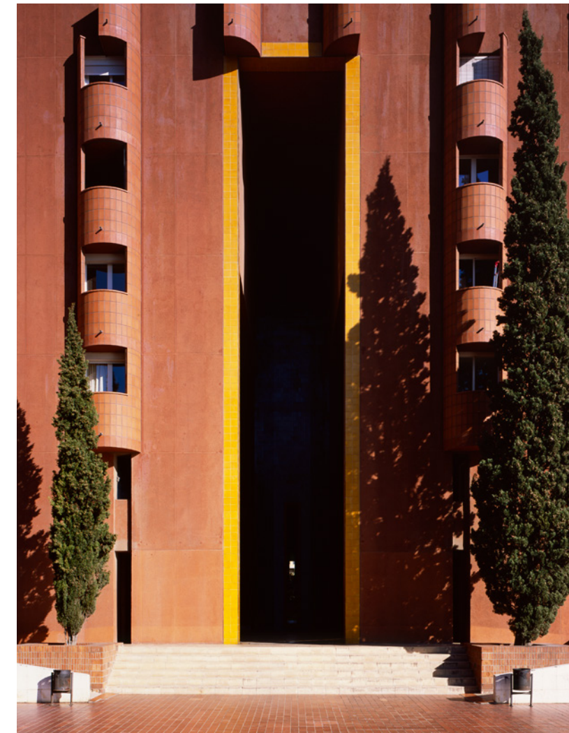
A dramatic entrance to the inner sanctum of the estate, bordered by cypress trees.
