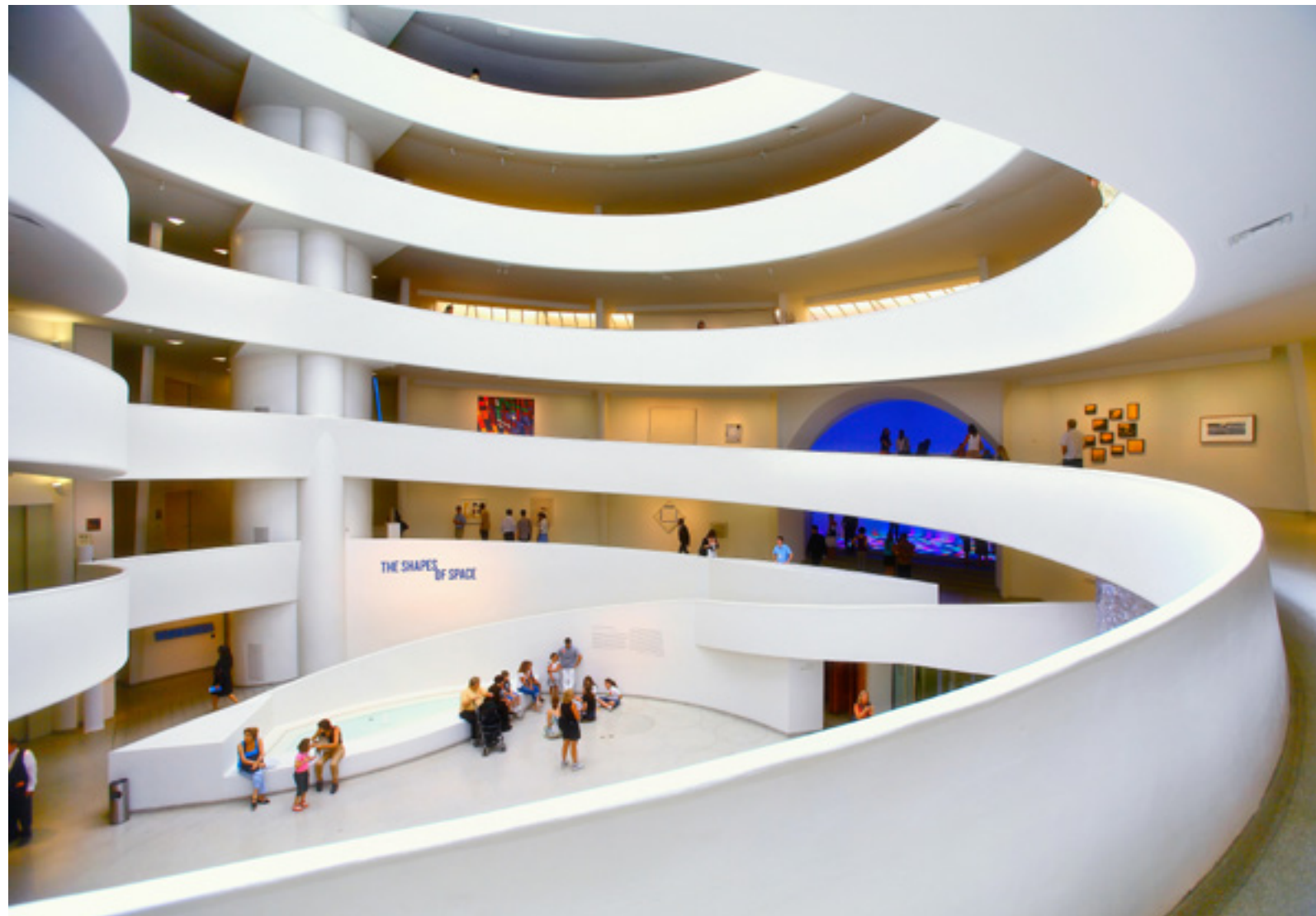
A quarter-mile of cantilevered concrete ramps climb the museum's outer walls. The building's domed skylight, or "oculus," consists of twelve sections resting on concrete structural columns that extend down through the building.
