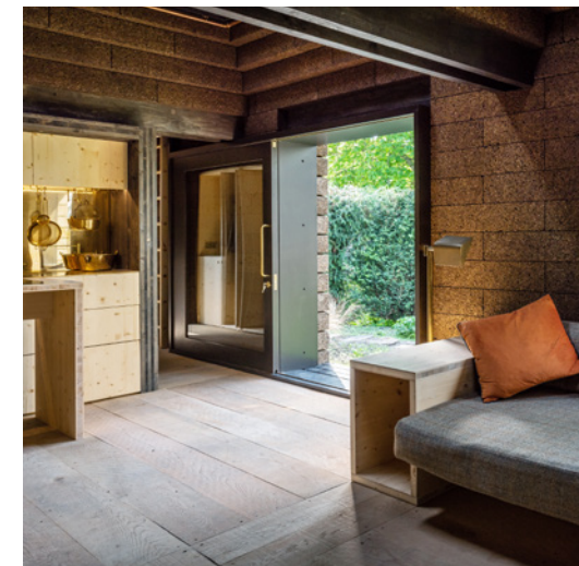
Opposite and above: The interior of the Cork House by Matthew Barnett Howland, Dido Milne, and Oliver Wilton. The house's monolithic walls and corbelled roofs are made almost entirely from solid, load-bearing cork.
